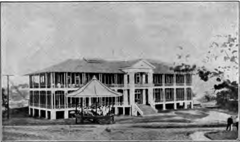
FIG. 10.— Club-house at Culebra, Panama, showing construction for thorough screening against mosquitoes.
